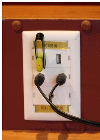
Or, if you are using a USB key, make sure it is plugged into a Patch Box USB port.
